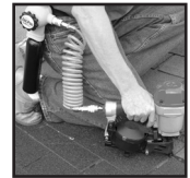
Roofing Shingle Installation
