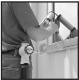
Window, Door, Bathroom Caulking
