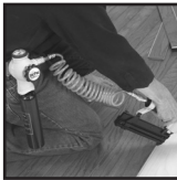
Hardwood Floor Installation
